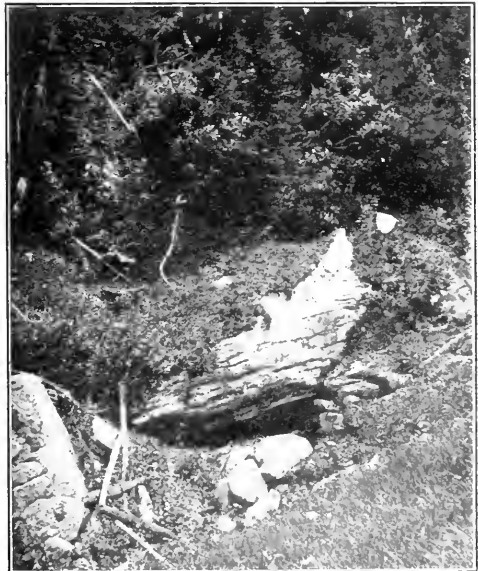
GOPHER BRIDGE, THE OLD ENTRANCE
